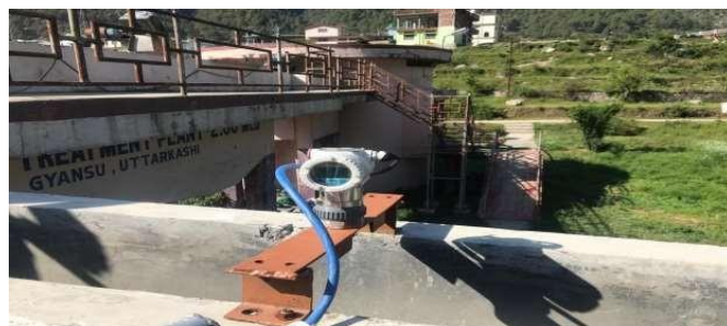
Fig.9 outlet from where the wastewater taken after the treatment of wastewater
