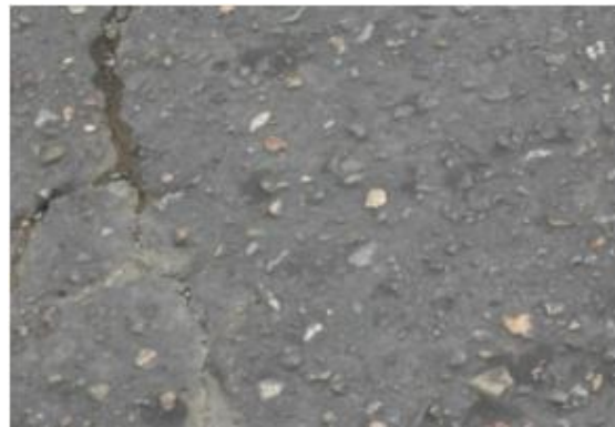
Figure 19. Pavement surface in H
