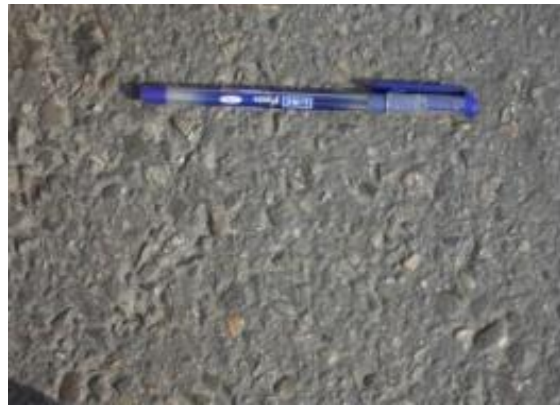
Figure 13. Pavement surface in B
