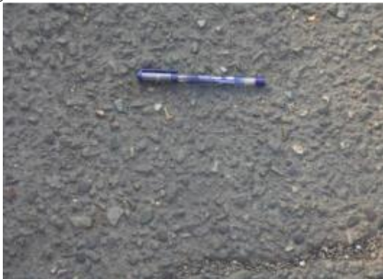
Figure 14. Pavement surface in C
