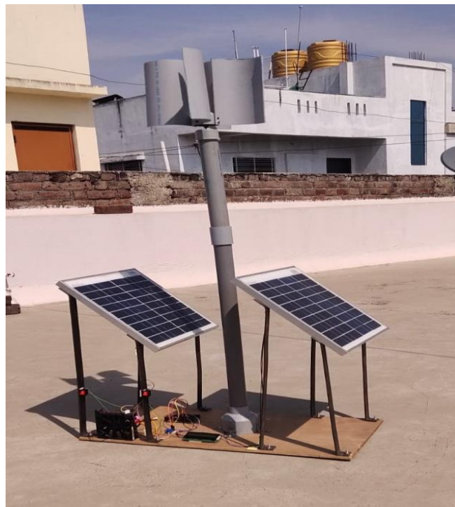
Fig2. Vertical Wind Turbine and Solar Hybrid System Experimental Setup
