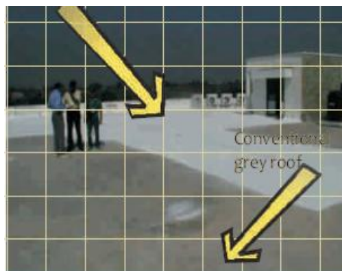
Figure 3 Third coat of Cool roof
