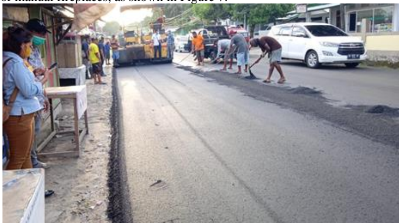
Figure 7 Method of Overlaying 1/2 of The Road
