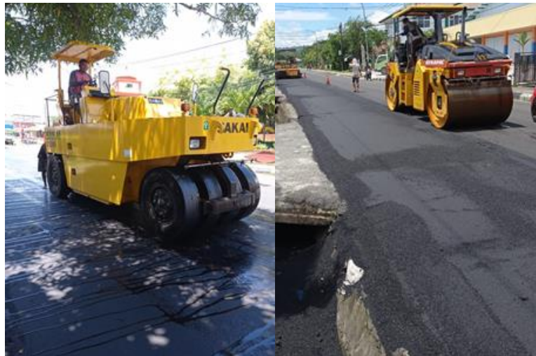
Figure 7 Pneumatic Tire Roller and Tandem Roller
