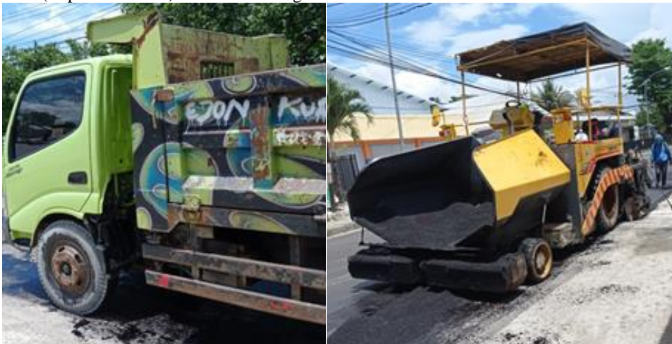
Figure 6 Dump Truck and Asphalt Finisher
