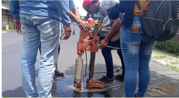
Figure 9 Core drill Sta. 1+900 (R) Laksdya Leo Wattimena Street
