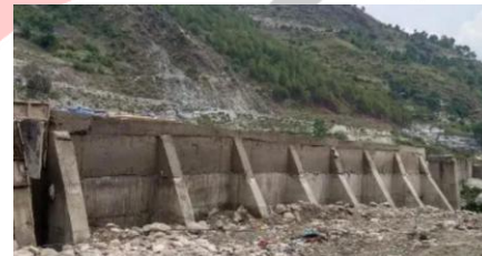
Fig 8 – R.C.C. Retaining wall
