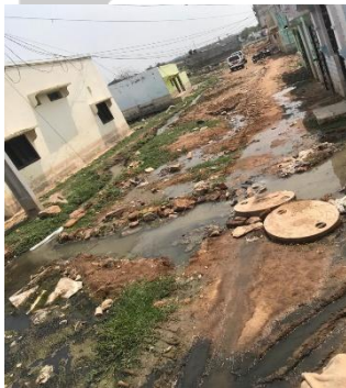
Fig 1 - Open Drainage and dumped garbage
