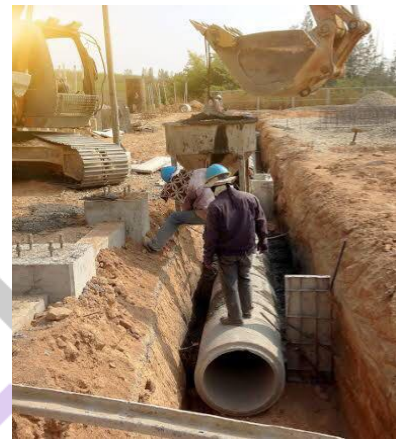
FIG 6- PIPE INSTALLATION
