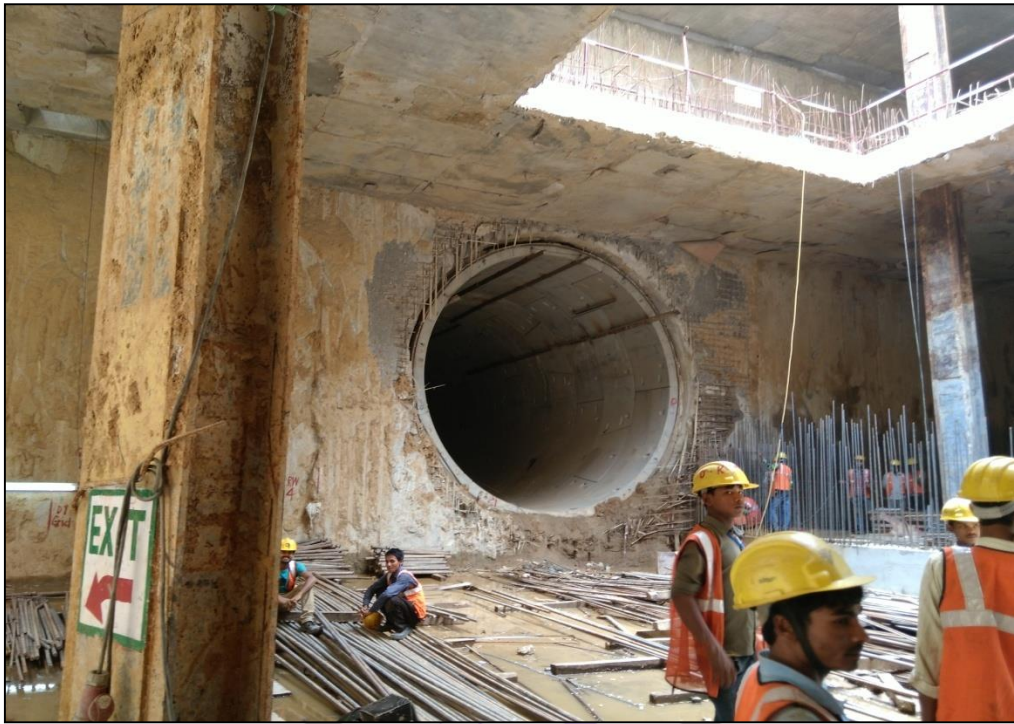
Tunnel at the site
