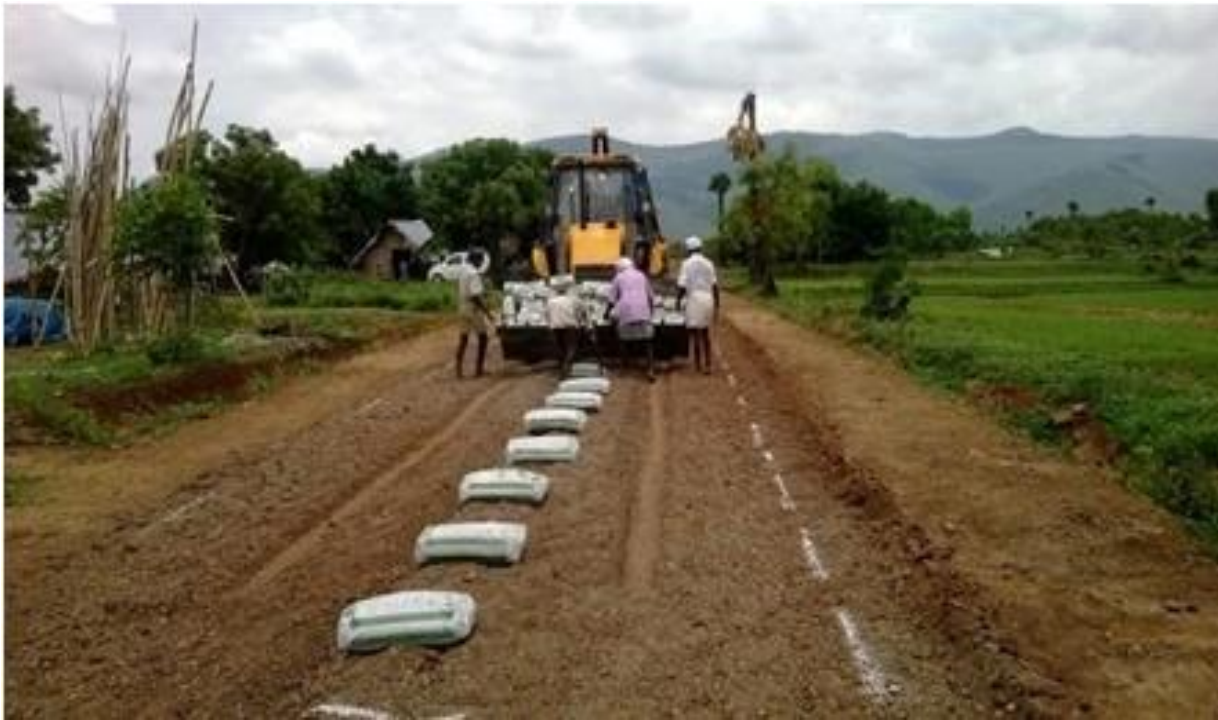
Fig. 2.5 Placing of RBI material in field
