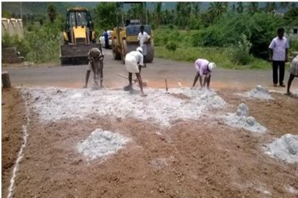
Fig. 2.6 Spreading of RBI Grade 81 material
