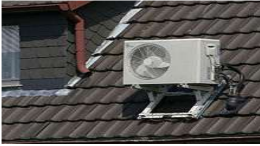
Figure 1.4.1.2 outside part of a ductless split-type air conditioner
