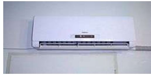
Figure 1.4.1.3 Indoor part of a ductless split-type air
