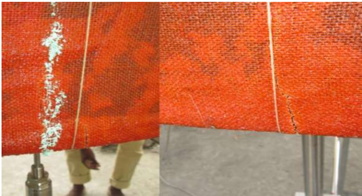
Fig – 6: Crack Formation in Contemporary Beam
