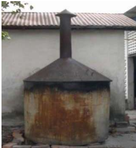
The ferro-cement furnace.
