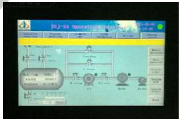
Fig 13: low vacuum sintering furnace condition before operation
