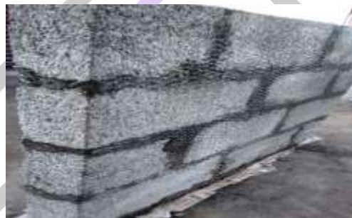
Figure 4 Confining of solid block walls
