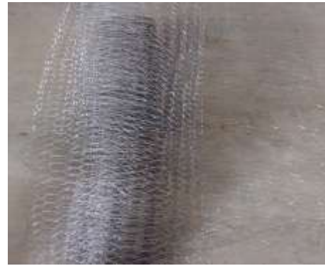
Figure 3 Casting of Wire Mesh
