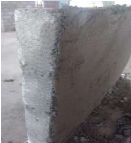
Figure 5 Plastering of Confined solid block masonry walls
