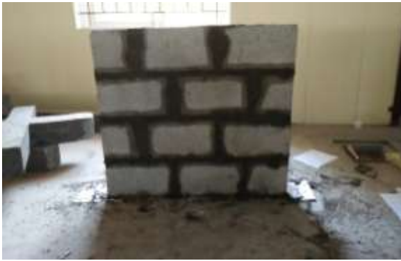
Figure 2 Casting of Solid Block Wall
