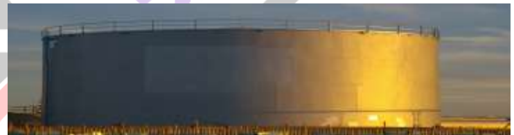
Fig1. Ground supported circular water tank
