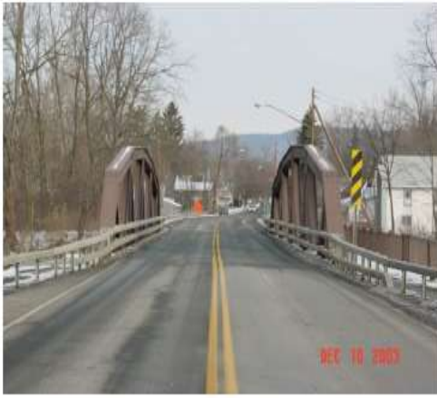
Fig.2 Roadway for Bentley Creek Bridge
