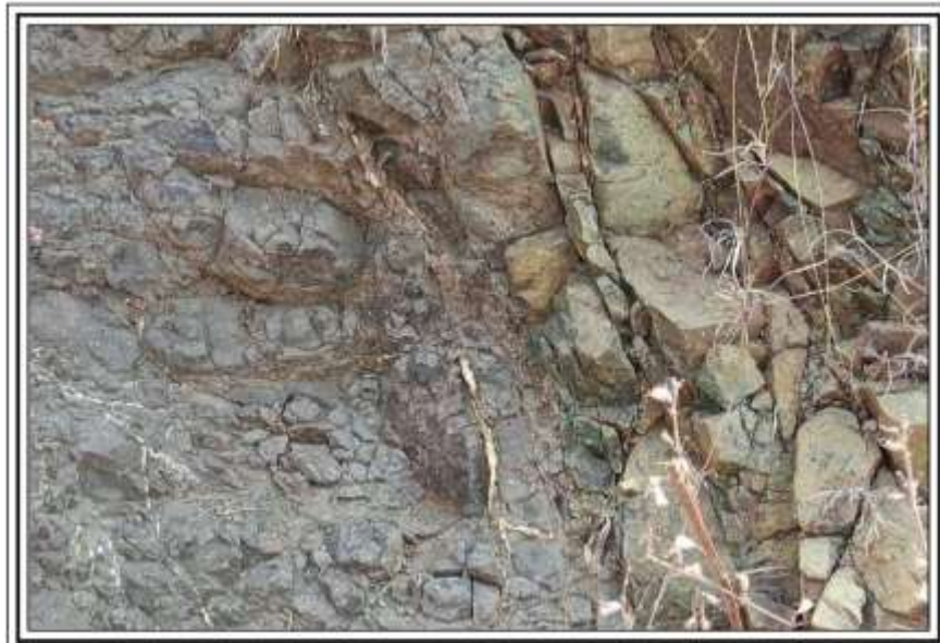
[Fig. 4 – Field photo of dyke close jointing here]
