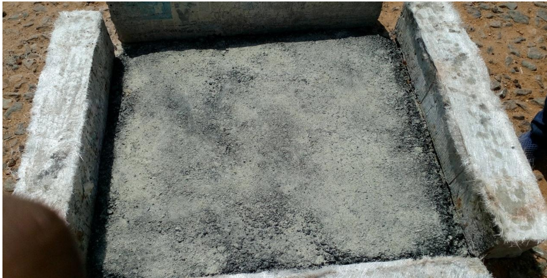
Fig. i. Road Laid To Our Project
